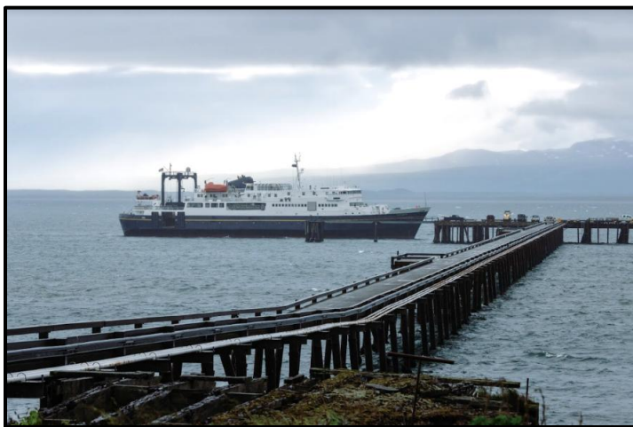
The work continues on multiple infrastructure projects throughout the region, including on the Cold Bay Dock.
