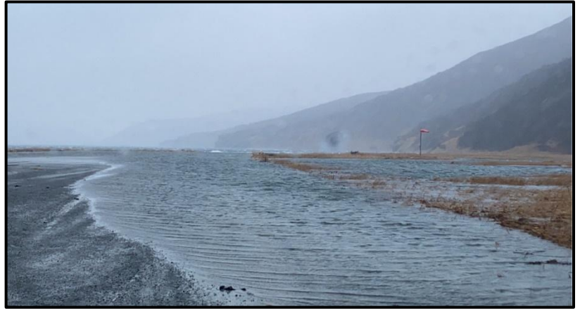
Flooding at the False Pass Airport due to a storm in December 2022.
