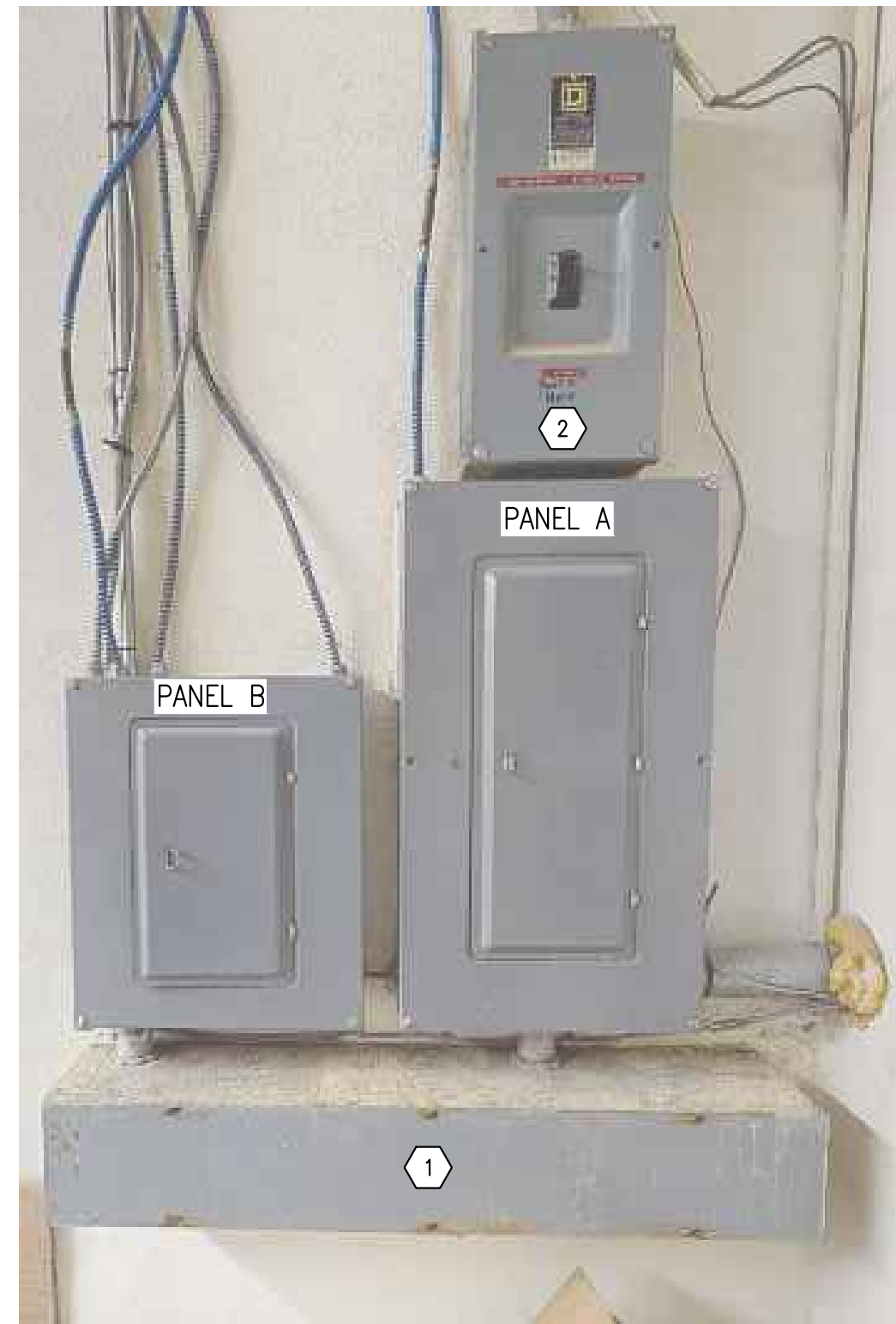
1 PHOTO - EXISTING PANELS E3.01 SCALE: NONE
