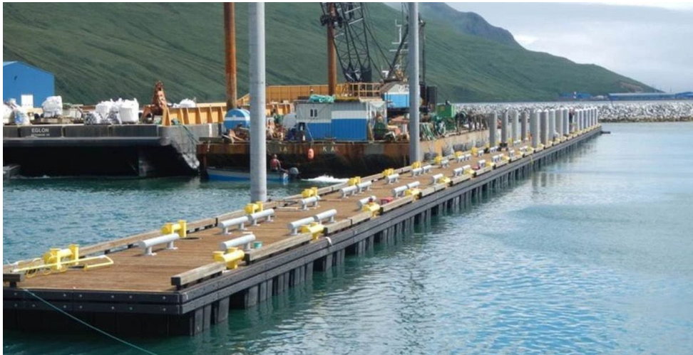
Figure 4. Akutan Harbor dock, Head of the Bay
