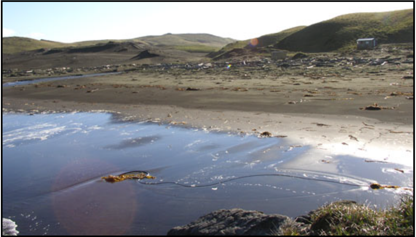
PHOTO 25: The road alignment is located behind the lower building, near the stream. This photo was taken from the breakwater near the proposed landing site, field site AN 83.
