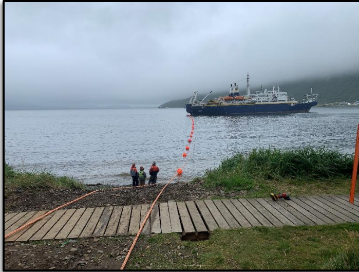
The c/s IT Intrepid (shown above in King Cove) began laying fiber optic cable during the summer from Unalaska to Kodiak, and to the south side of the Alaska Peninsula as part of GCI's AU-Aleutians Project. Photo courtesy: GCI.
