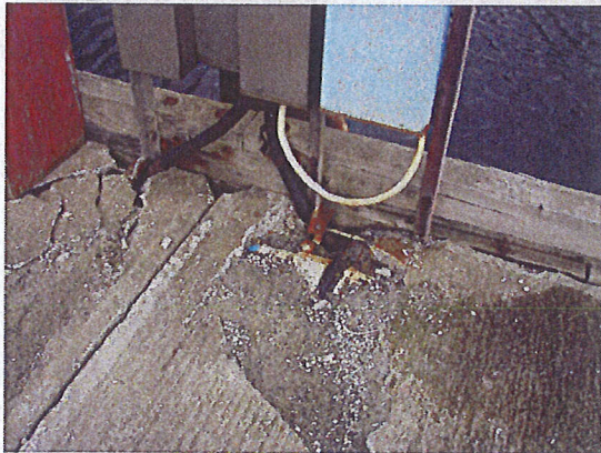
Deck delaminating at electric pedestal
