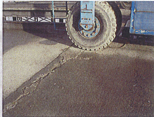
Concrete damage at approach
