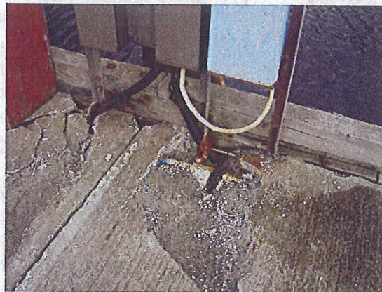
Deck delaminating
