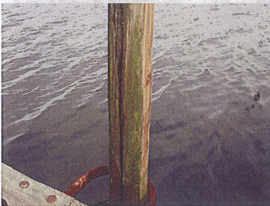
Deteriorated timber pile
