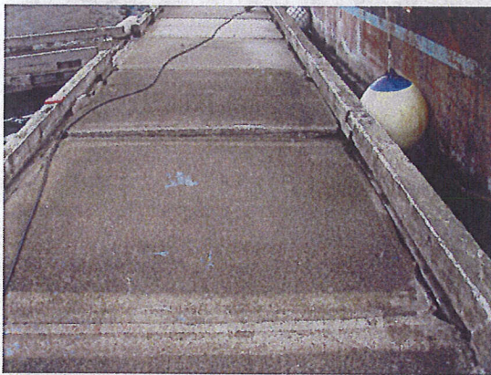
Loose concrete modules
