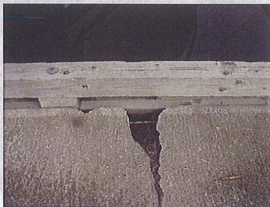
Spalled deck
