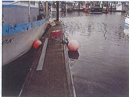
Listing finger with low freeboard
