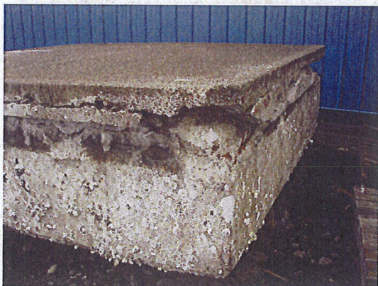
Concrete float with damage below the deck
