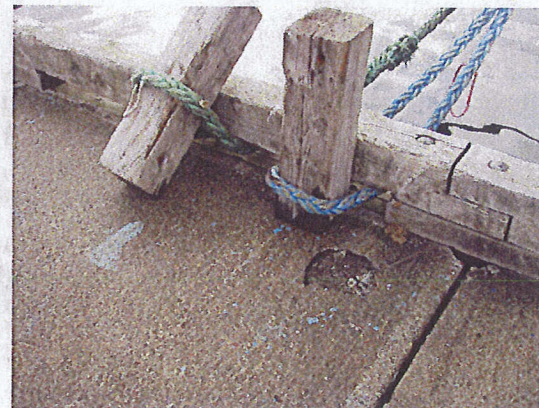
Deck damage at mooring toggle
