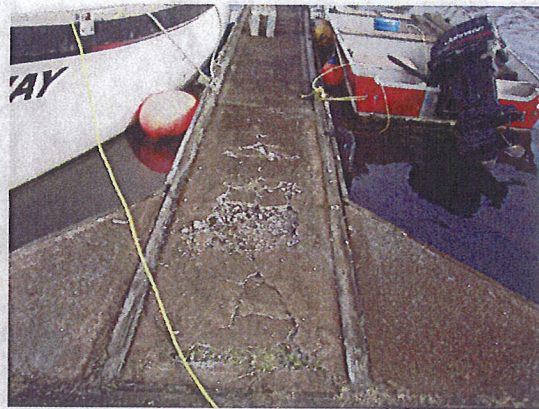
Spalled deck
