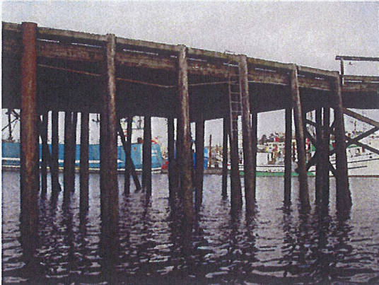
Timber fenders and ladder
