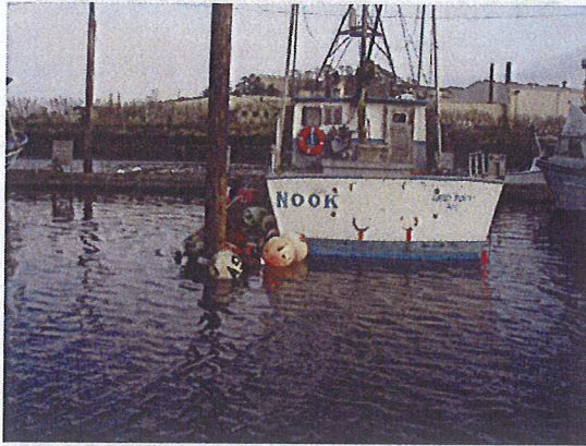
Listing and sinking finger
