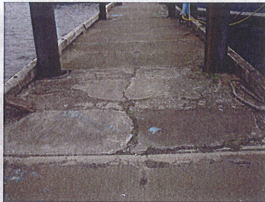
Delaminating deck
