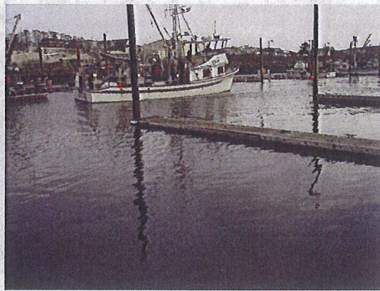
Finger with Low Freeboard and listing
