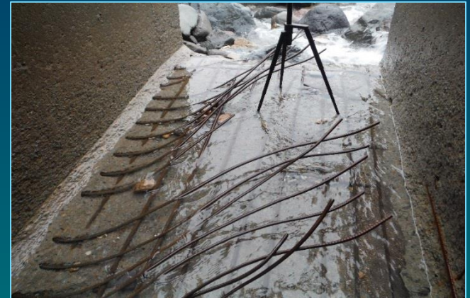
Concrete Structure Eroding
