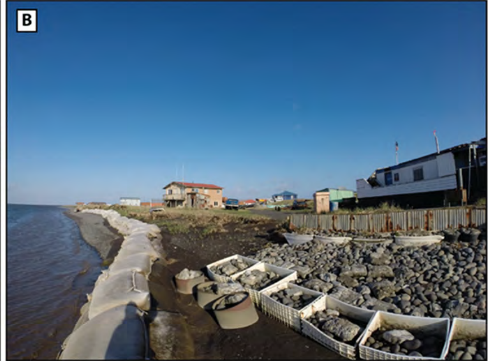
Figure 27. Seawall and sediment containers in place along the lagoon coastline of Nelson Lagoon. May 2019, UAF-ACGL.
