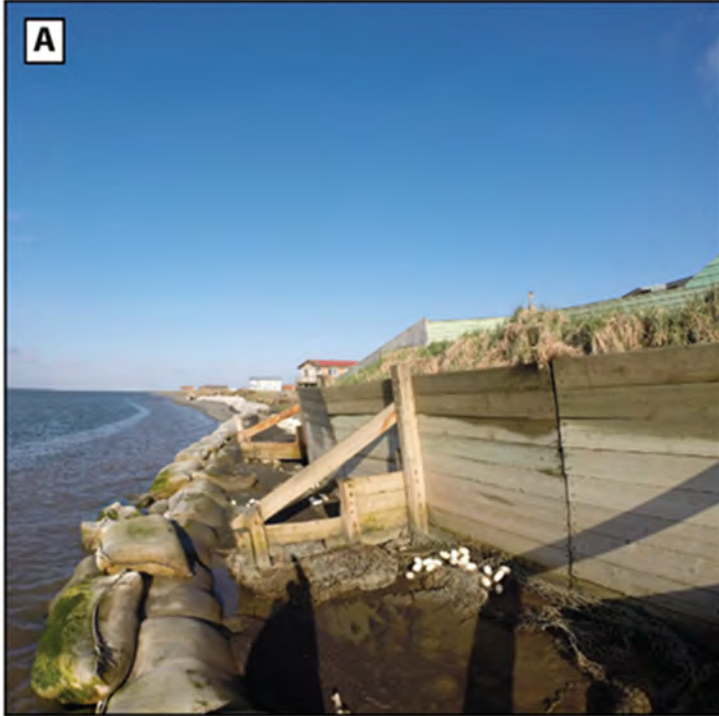
Figure 27. Seawall and sediment containers in place along the lagoon coastline of Nelson Lagoon. May 2019, UAF-ACGL.
