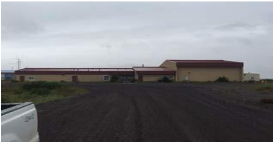
Cold Bay School-Front of Building
